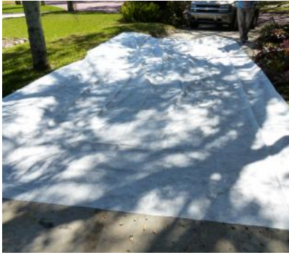
1. Lay out full 12-foot width.
